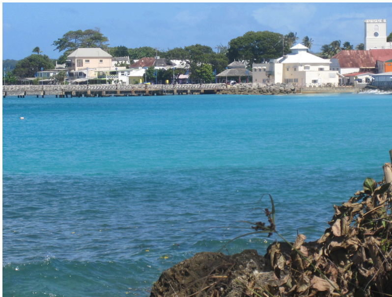
Photo 3: Section to north showing existing jetty.
