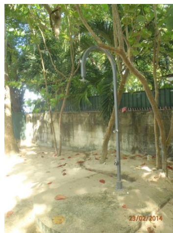
Figure 5.34: Public shower facilities
